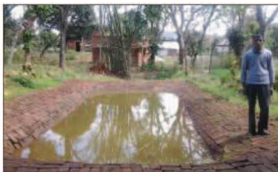
Demonstration of water harvesting structure developed under NICRA
